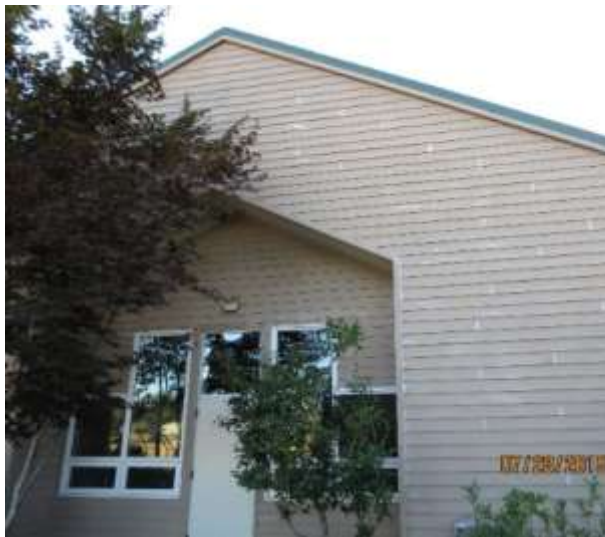
Completed Surface Preparation July 28, 2015
