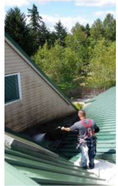
Power Washing the North Sanctuary Wall
